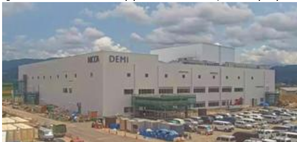
Figure 50. Fukui Smart Factory (Under Construction, as of July 29)
