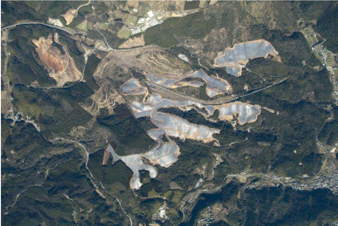
Figure 13. CS Hiji-machi Dai-Ni Power Plant (Oita, 54 MW)
